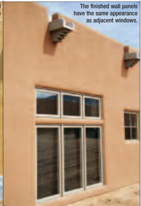
The outside masonry surface is painted a dark color before the windows are installed to increase heat absorptency.
